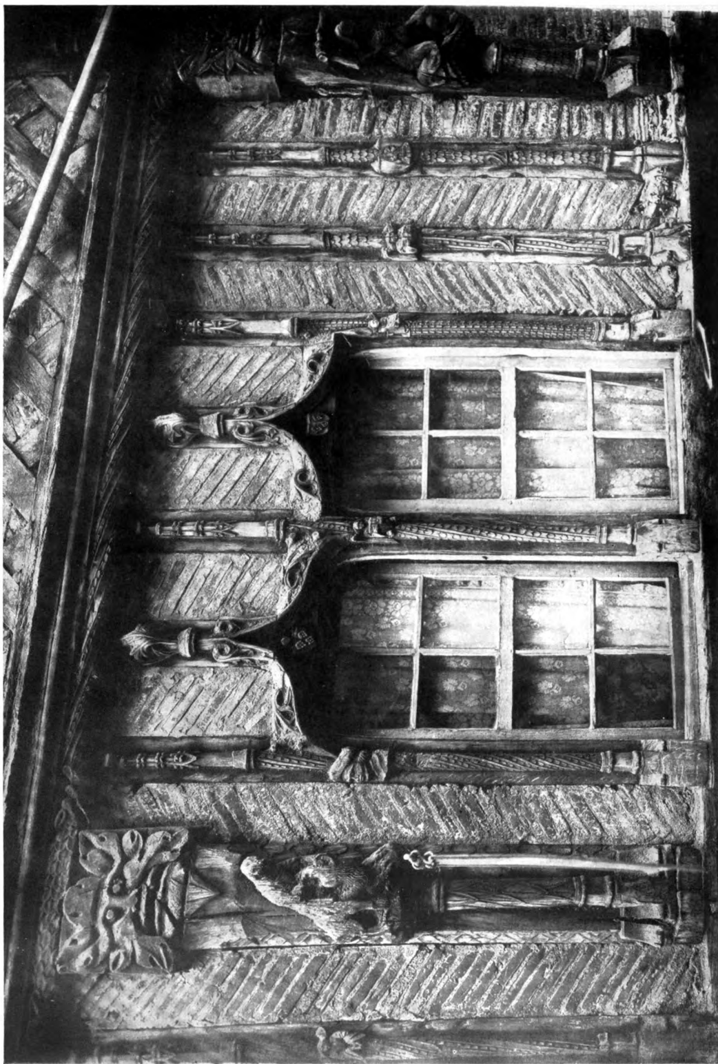
Lisieux (Calvados) . . Francis the First House, XVth Century, showing the details of woodwork
