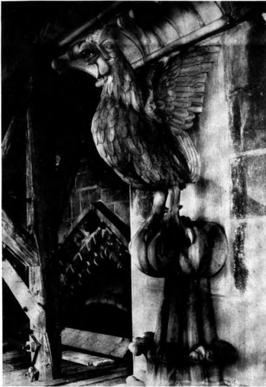
Reims (Marne) (Lead Work) Cock
