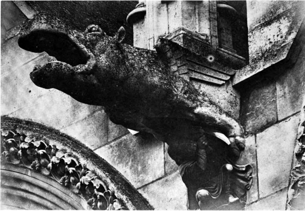
Laon Cathedral (Aisne) Restored
