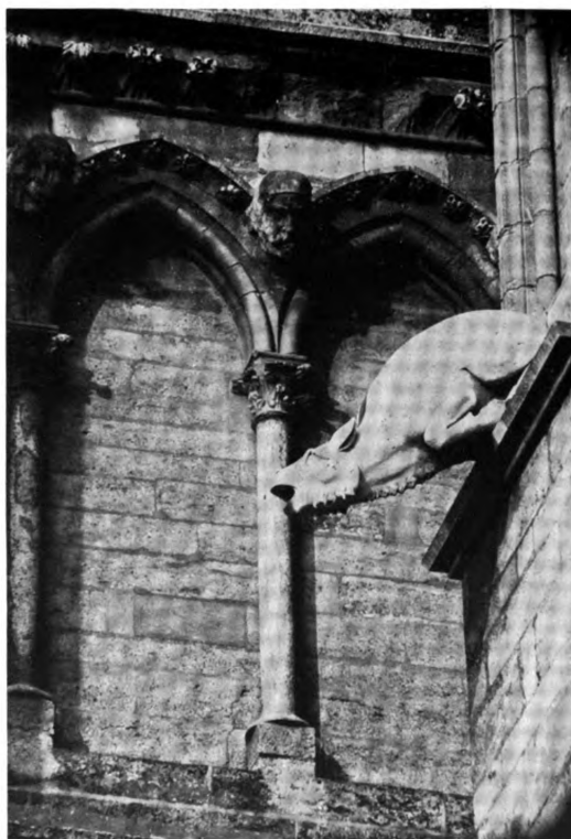
Reims Cathedral (Marne) North Side
