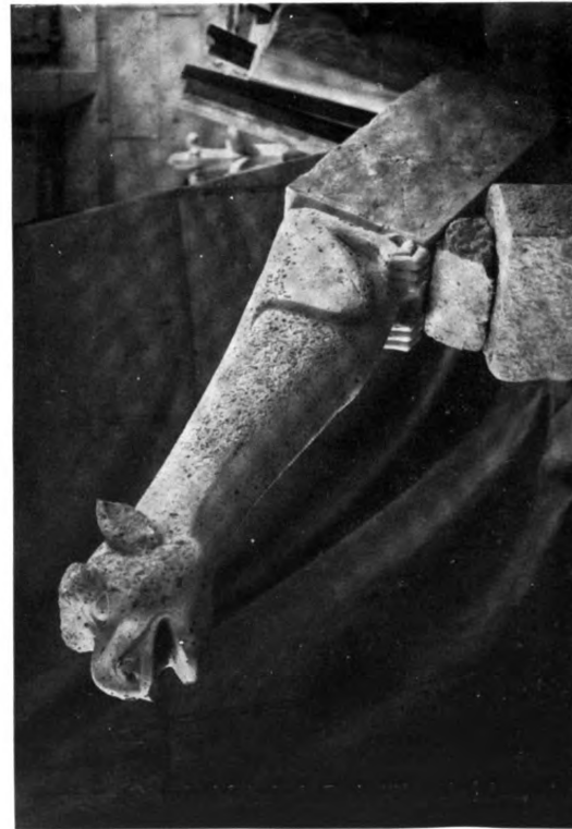
Soissons (Aisne) Restoration South Nave
