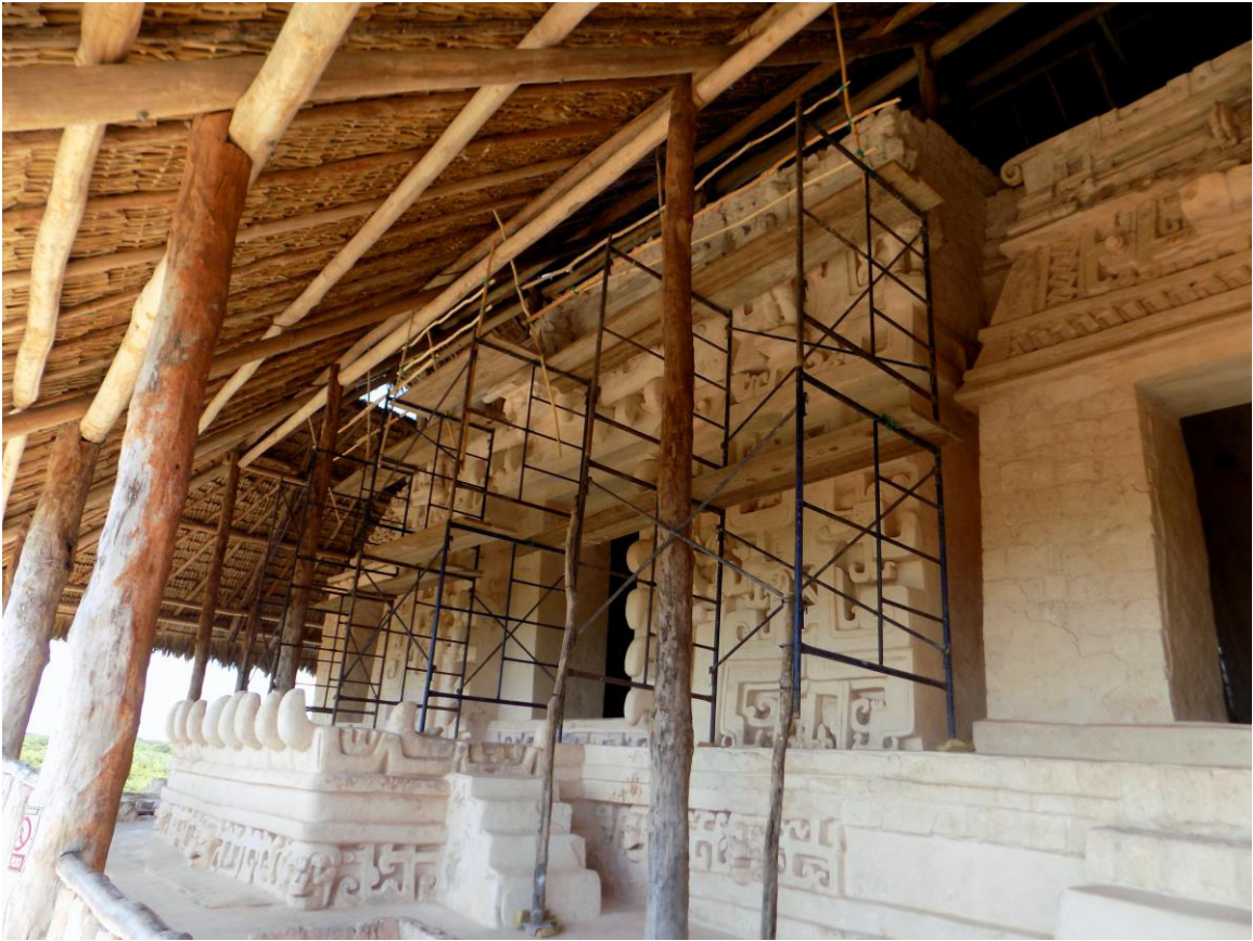
Figure 1.4 The façade of Room 35, Structure 1, Ek' Balam (Photo by author: 10/2015)
