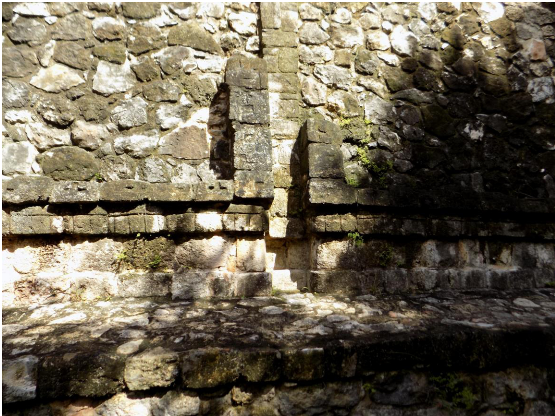
Figure 3.26 Visual dislocation of the lower range-type structure, GT-1, Ek' Balam (Photo by author: 10/2015)
