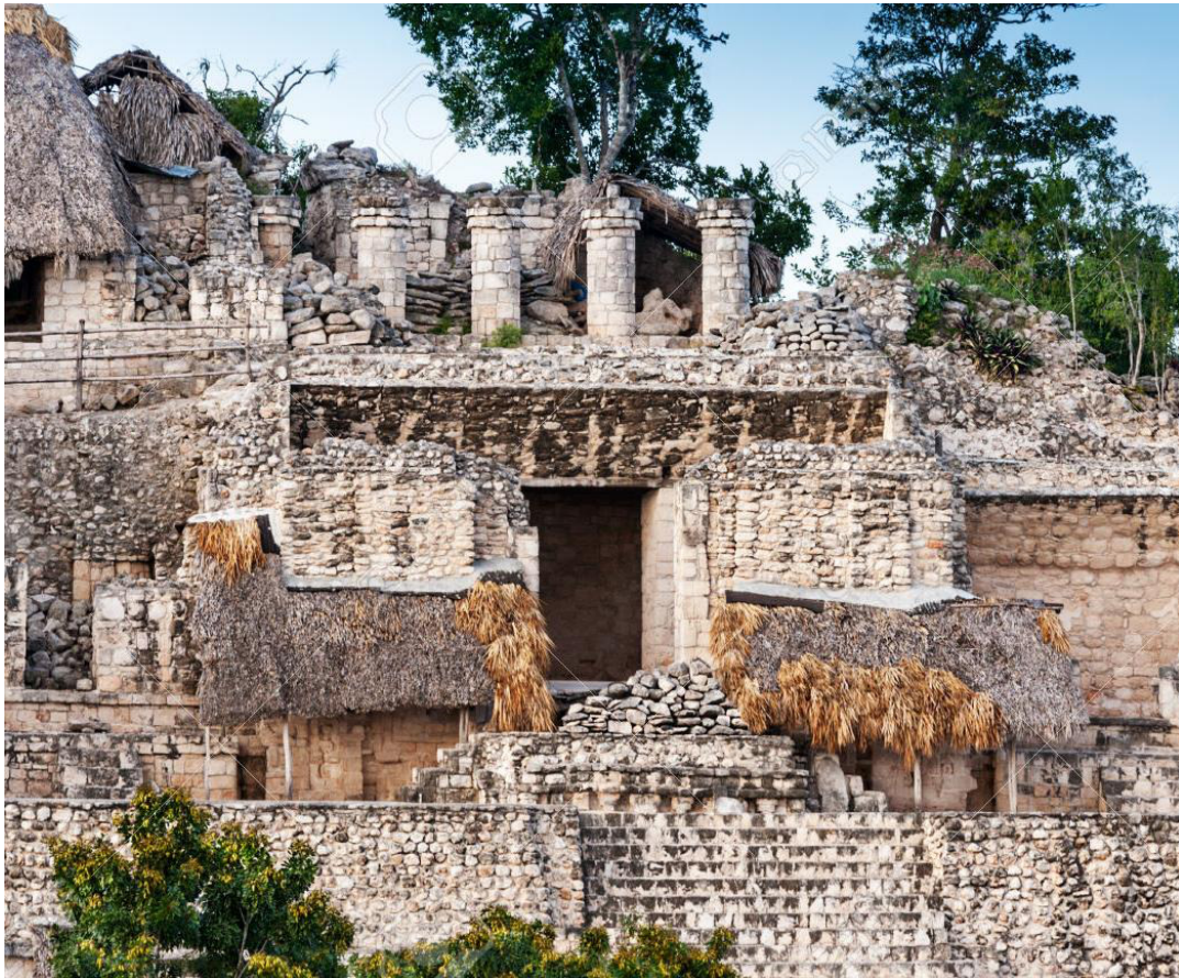
Figure 1.9 The façade of Room 29, Structure 1, Ek' Balam (Photo by author: 10/2015)
