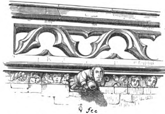
Parapet, Brailes Church, Warwickshire.
